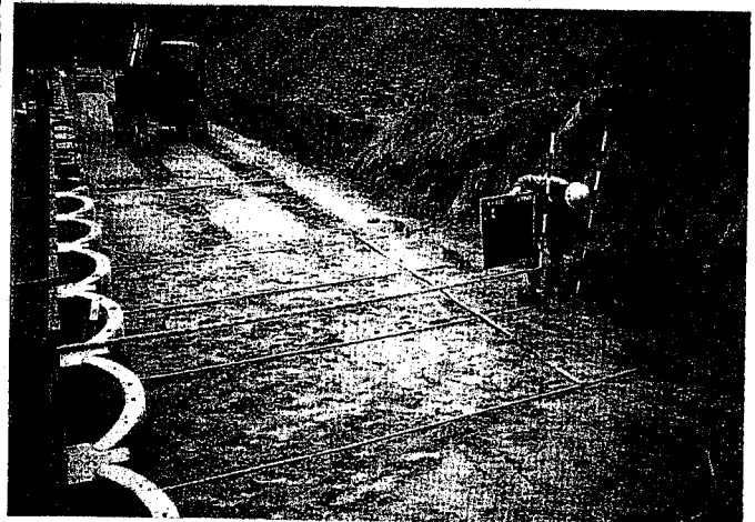
Photo 1 Setting of arch wall
